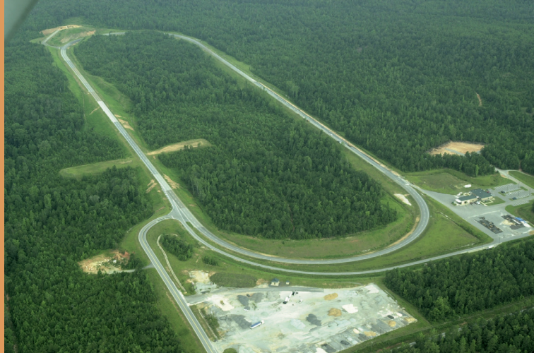
IMAGE A: GlasGrid was installed at the National Center for Asphalt Technology (NCAT) pavement test track in Opelika, AL.
